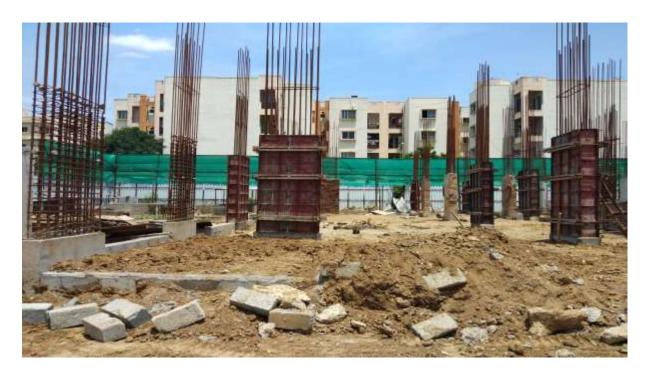
In Block D3, Shuttering and Bar bending Works for First half of Second floor level on Progress
