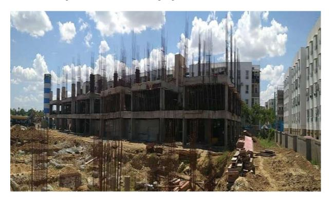
In Block B2 Excavation Work for Pile Cap Works & Barbending work for Pile Cap on process.
