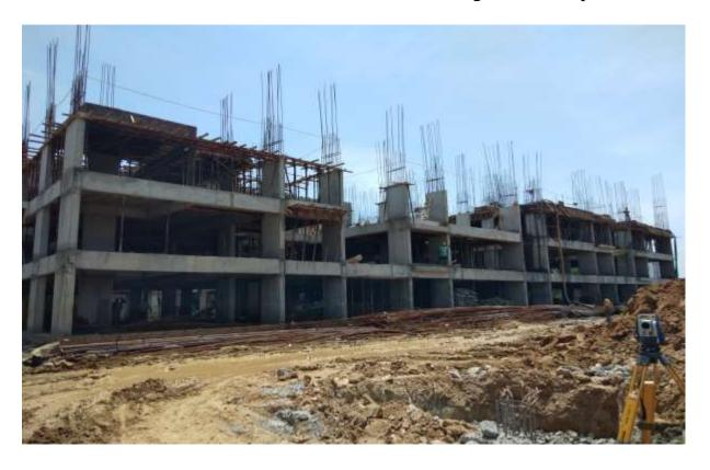
In Block D2 Shuttering & Barbending Works for Third Floor Level Slab on progress.
