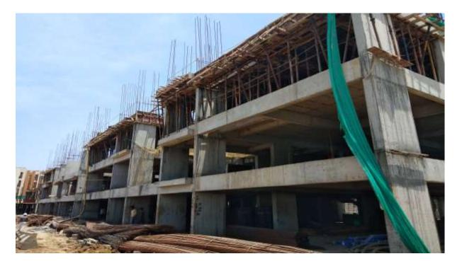
In Block D3 , Column Concrete upto Stilt floor & Backfilling on Progress for Second half of the Block
