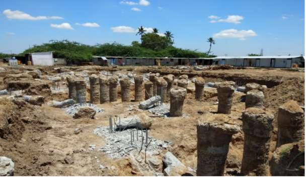
In Block A2 Excavation works, PCC Work, Pile chipping work in progress.
