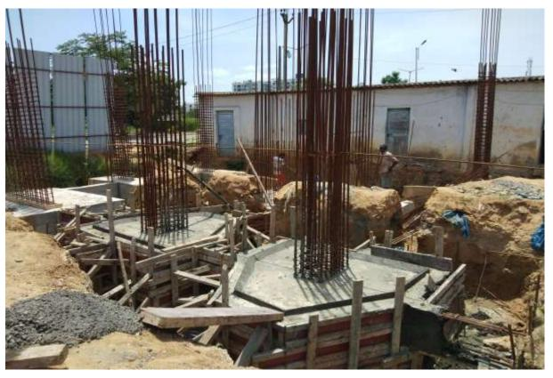
In Block A1 Excavation works , PCC Work, Pile Chipping work in progress.
